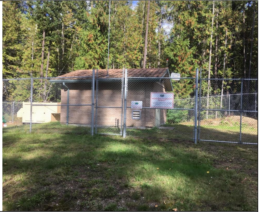
Well Pump House
